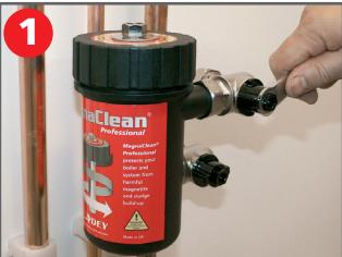
**Important** – Before commencing any servicing work, turn off the electrical supply to the boiler. Turn off both isolation valves to the marked OFF position. Loosen the air vent to release internal pressure. When venting, protect the surface below the canister with a dust sheet or container to capture any drops of water.
