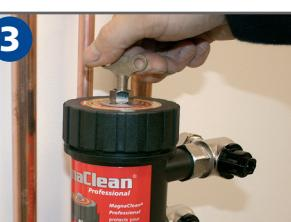
Replace the Pro-Fill air vent. Allow the system to circulate for 30 seconds. Open the Pro-Fill screw two turns and back flush until clear.
