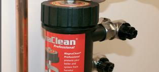
Remove the complete lid assembly from the *MagnaClean Professional*. Turn the lid assembly upside down in order that the underside of the lid acts as a drip tray.
