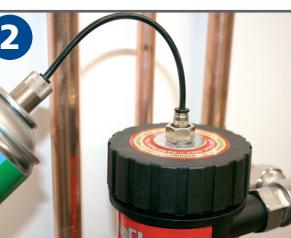
Wait for five seconds before removing the adaptor. The Pro-Fill air vent will accept all market-leading chemicals in either liquid or concentrate form.
