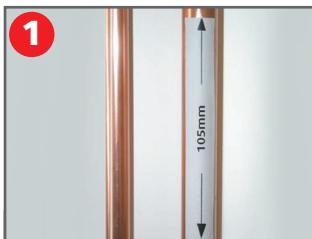
Drain the central heating system or plug-off feed and expansion tank and release the system pressure. Measure and mark a 105mm section for a 22mm unit and a 190mm section for a 28mm unit when making the connections with elbows as shown.
