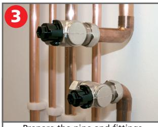
Prepare the pipe and fittings accordingly. Lubricate the olives and assemble the valves on the pipe, hand tighten.
